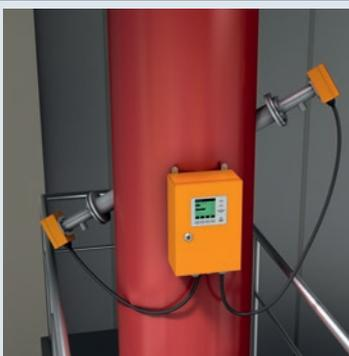
Steam flow measurement often requires compromise, but it doesn't have to. Ultrasonic flowmeters operate around the world on challenging high-value steam flow installations. These include custody transfer of steam where accuracy is important for billing, loss of pressure can be avoided or bi-directional flow needs to be measured.
