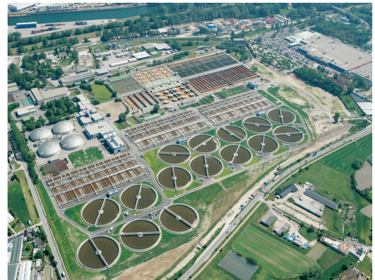
Figure 1, wastewater treatment plant. This treatment plant receives wastewater from a network of lift stations, each of which must be controlled and monitored to assure correct operation.
